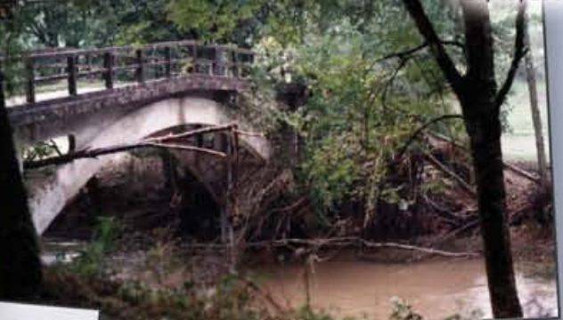
Passerelle de Chambon Veyrinas (Briance) 23/09/1993
